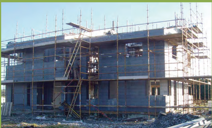
Two Storey Construction
