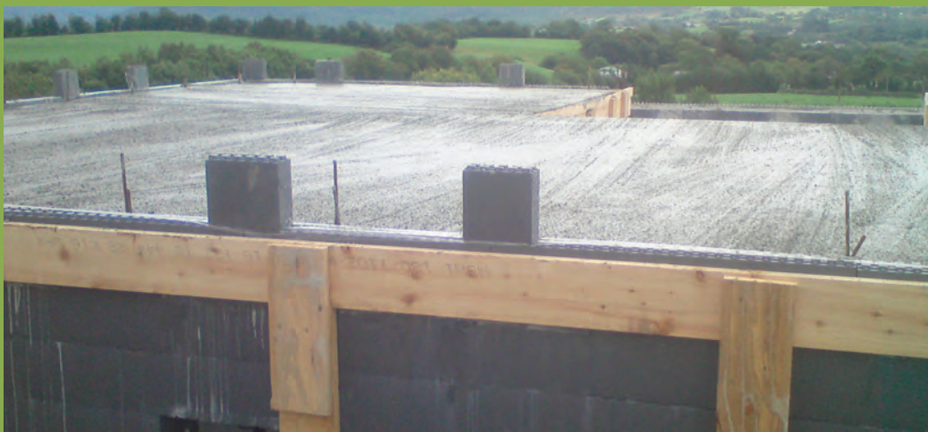
Shuttering to edge of floor and concrete pour
