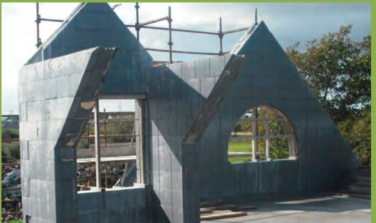
First Floor Dormer Window and Gable Wall Construction
