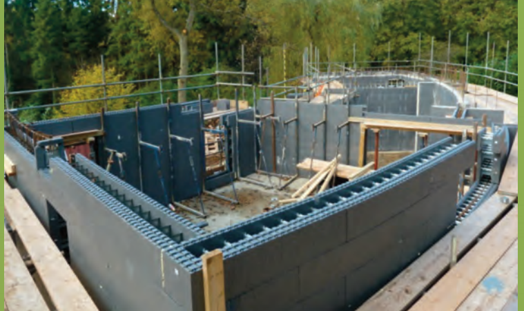
ICF Curved Wall Construction
