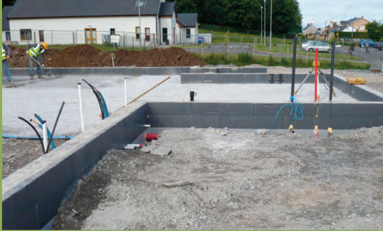
Thermohouse ICF Rising Walls / Dead Work
