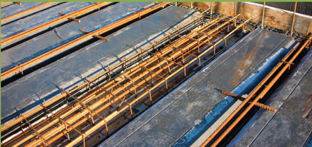
Typical Floor Installation with insitu beam
